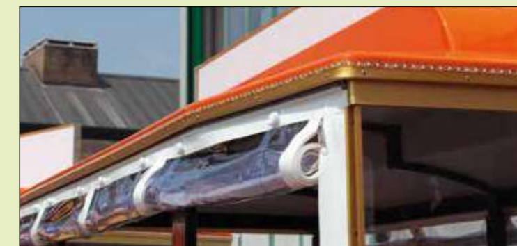
Decorative led lighting system around roof
